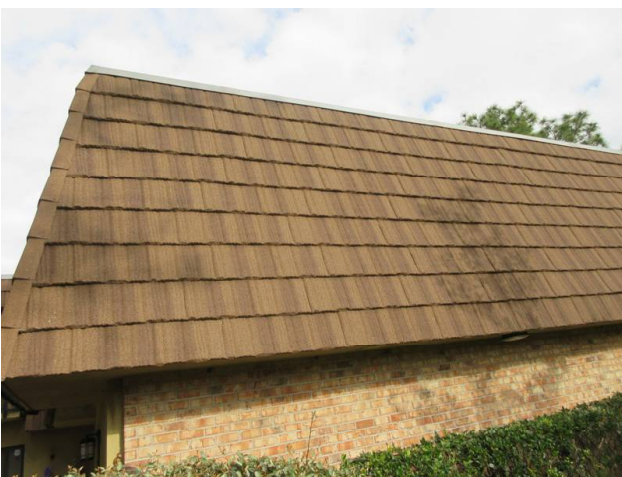
MANSARD WALLS REPLACED 2018
