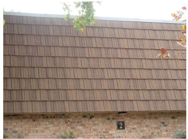
MANSARD WALLS REPLACED 2018
