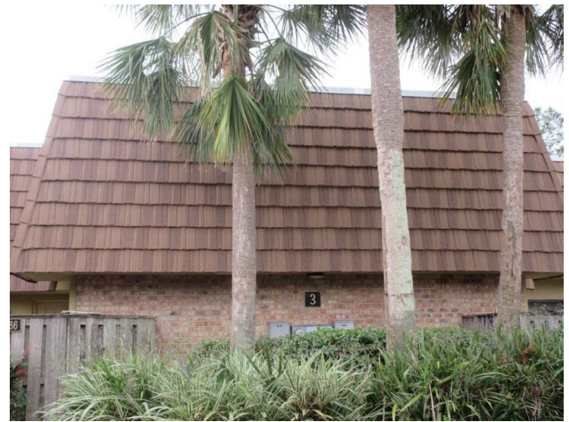
MANSARD WALLS REPLACED 2018
