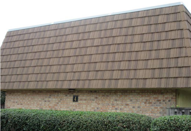
MANSARD WALLS REPLACED 2018
