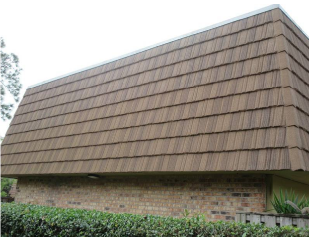
MANSARD WALLS REPLACED 2018
