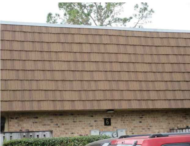
MANSARD WALLS REPLACED 2018
