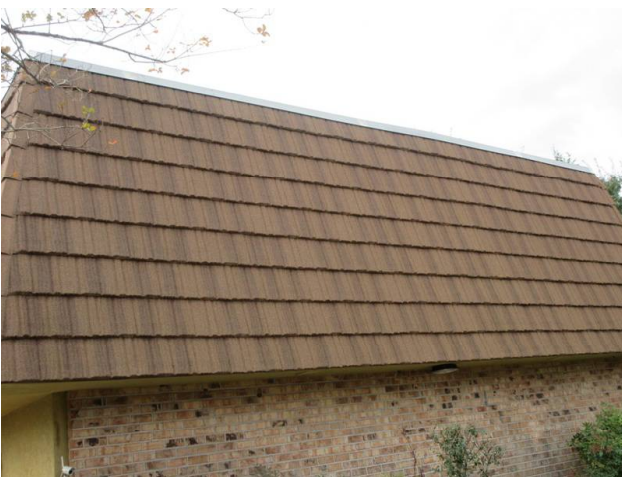
MANSARD WALLS REPLACED 2018
