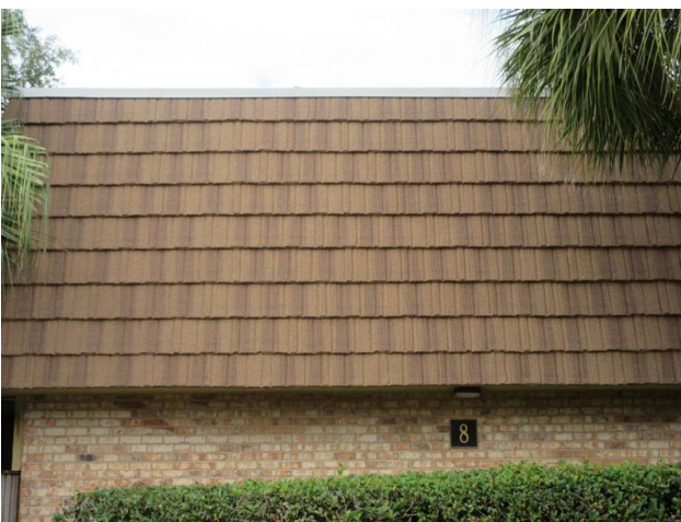
MANSARD WALLS REPLACED 2018
