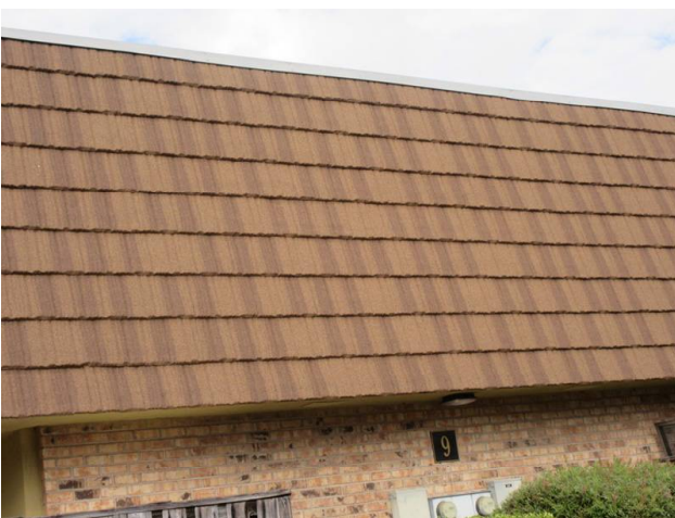
MANSARD WALLS REPLACED 2018
