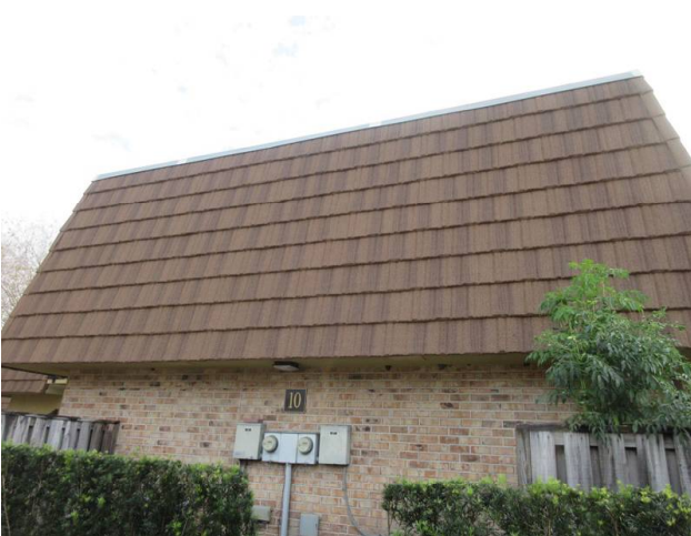
MANSARD WALLS REPLACED 2018
