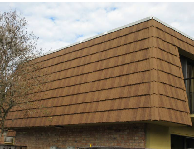
MANSARD WALLS REPLACED 2018
