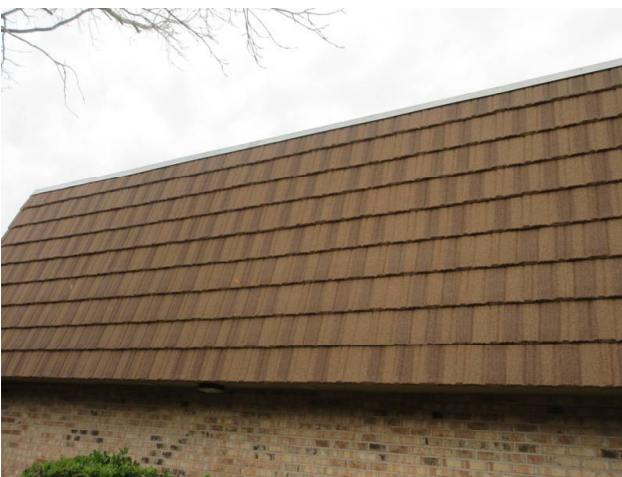
MANSARD WALLS REPLACED 2018
