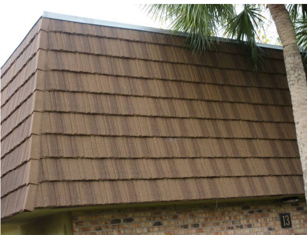
MANSARD WALLS REPLACED 2018
