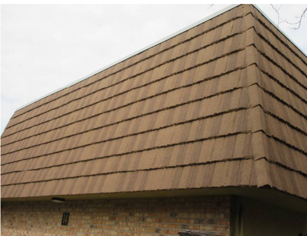
MANSARD WALLS REPLACED 2018
