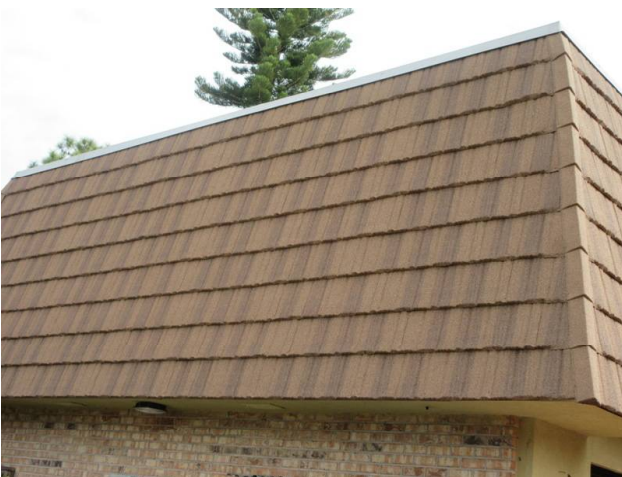
MANSARD WALLS REPLACED 2018
