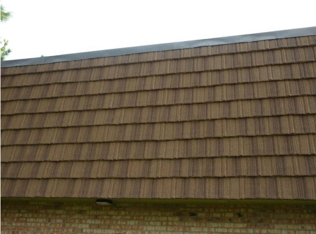
MANSARD WALLS REPLACED 2018
