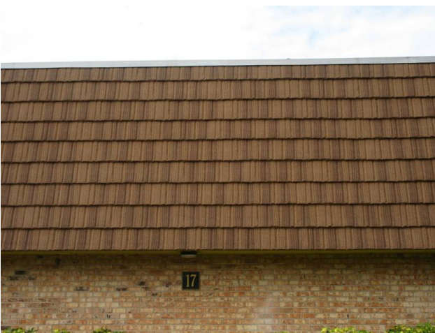
MANSARD WALLS REPLACED 2018
