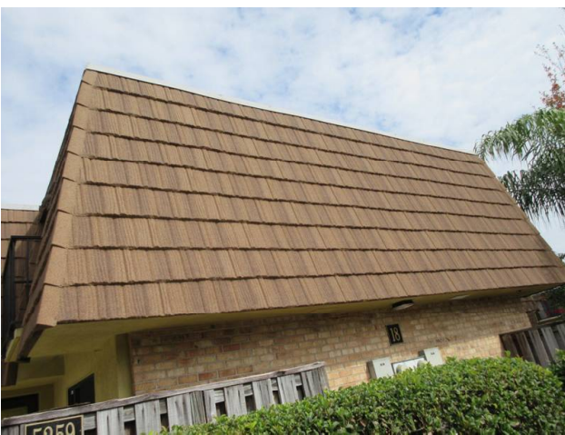
MANSARD WALLS REPLACED 2018
