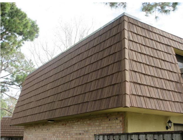
MANSARD WALLS REPLACED 2018
