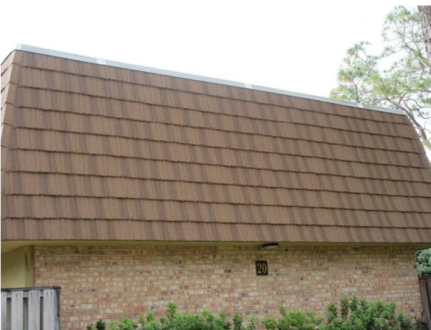
MANSARD WALLS REPLACED 2018
