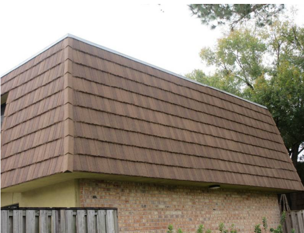
MANSARD WALLS REPLACED 2018
