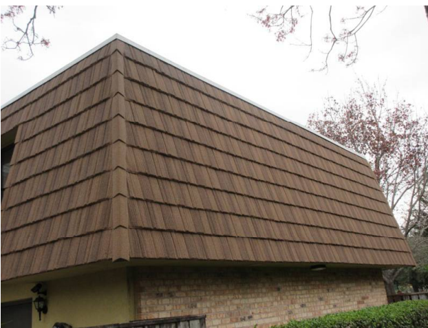
MANSARD WALLS REPLACED 2018
