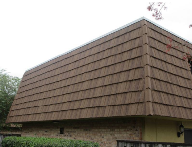
MANSARD WALLS REPLACED 2018
