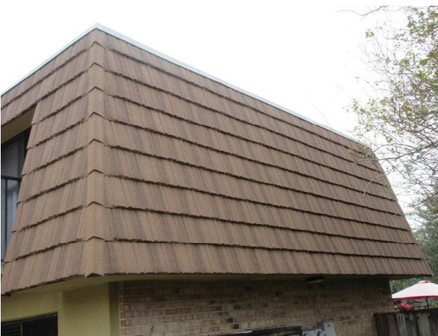
MANSARD WALLS REPLACED 2018
