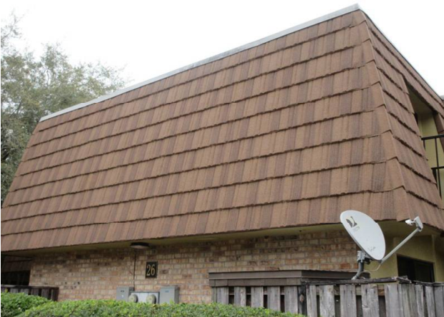
MANSARD WALLS REPLACED 2018
