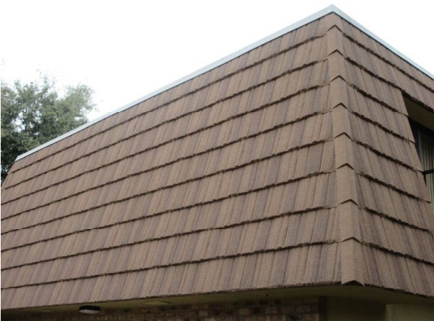
MANSARD WALLS REPLACED 2018
