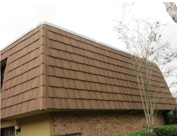
MANSARD WALLS REPLACED 2018
