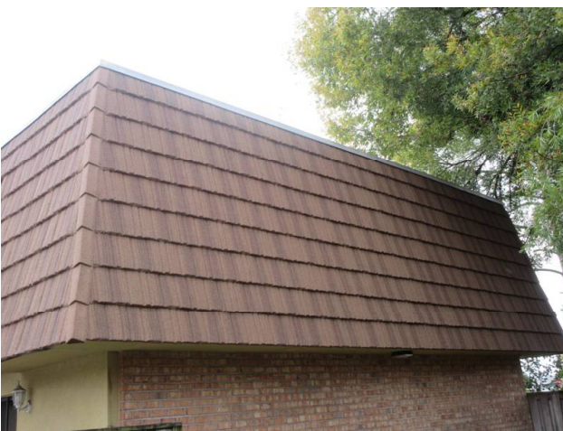
MANSARD WALLS REPLACED 2018
