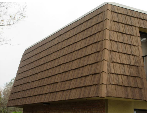
MANSARD WALLS REPLACED 2018
