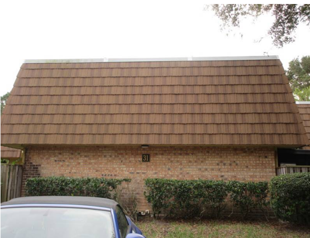
MANSARD WALLS REPLACED 2018
