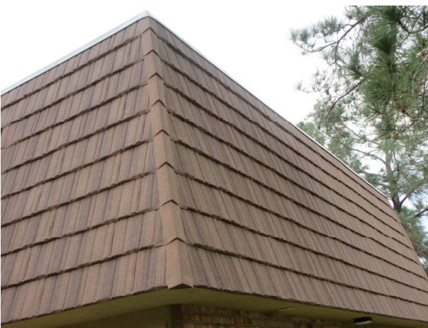
MANSARD WALLS REPLACED 2018
