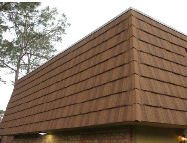
MANSARD WALLS REPLACED 2018
