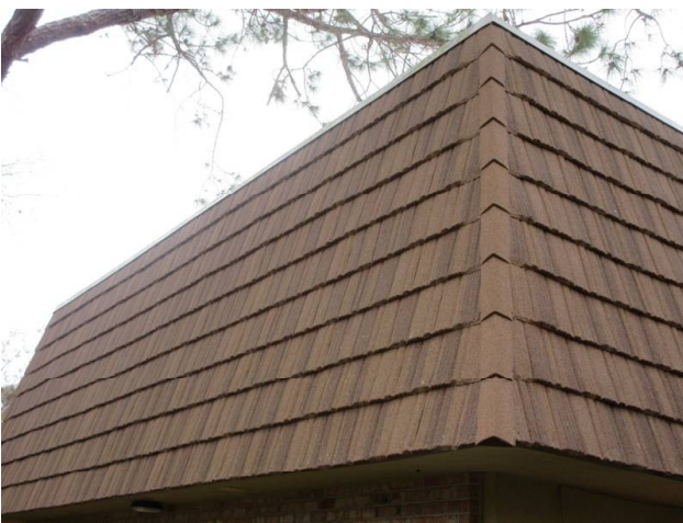
MANSARD WALLS REPLACED 2018
