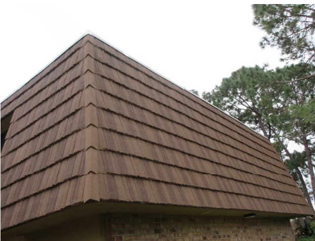
MANSARD WALLS REPLACED 2018
