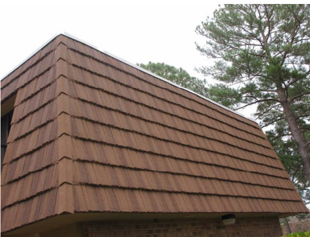
MANSARD WALLS REPLACED 2018
