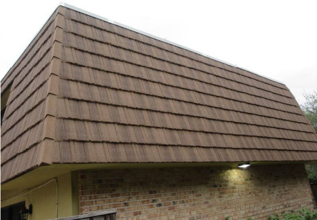
MANSARD WALLS REPLACED 2018
