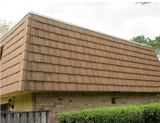
MANSARD WALLS REPLACED 2018
