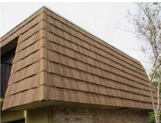
MANSARD WALLS REPLACED 2018
