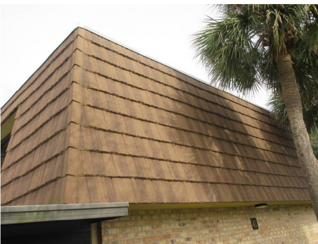
MANSARD WALLS REPLACED 2018
