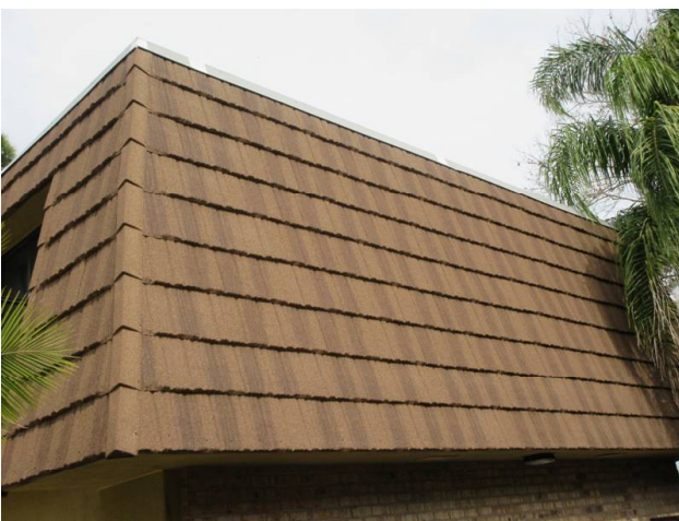
MANSARD WALLS REPLACED 2018
