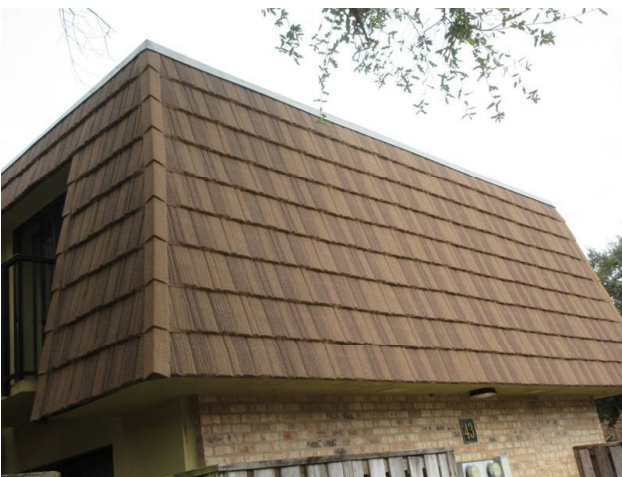
MANSARD WALLS REPLACED 2018
