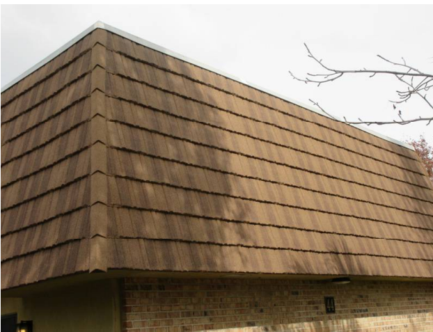
MANSARD WALLS REPLACED 2018
