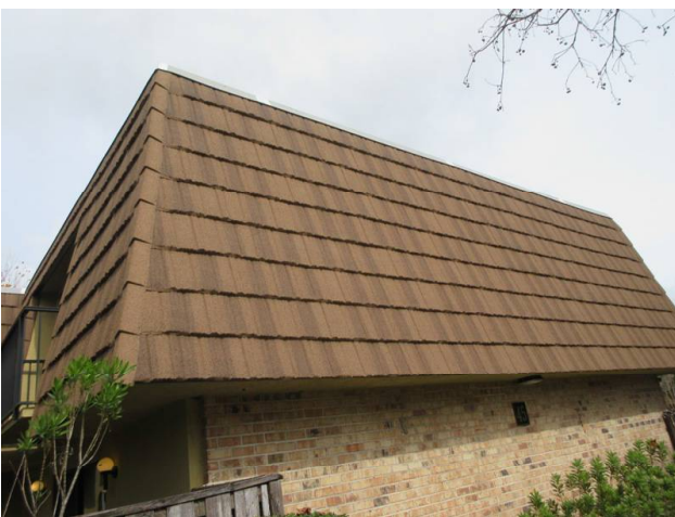
MANSARD WALLS REPLACED 2018
