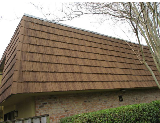
MANSARD WALLS REPLACED 2018
