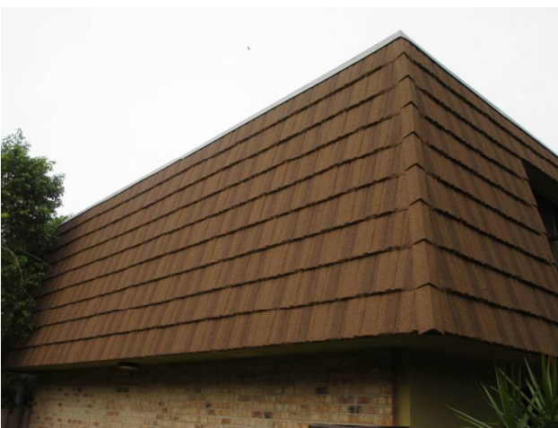
MANSARD WALLS REPLACED 2018
