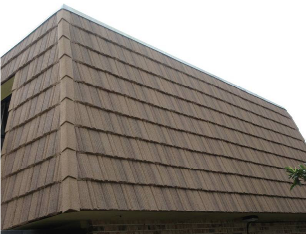
MANSARD WALLS REPLACED 2018
