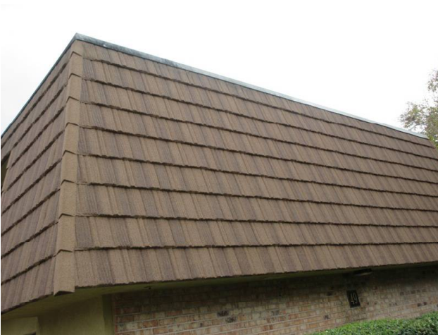
MANSARD WALLS REPLACED 2018
