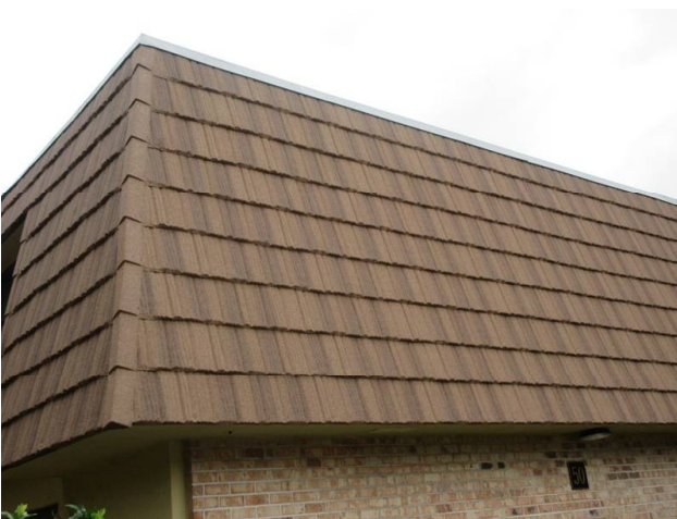
MANSARD WALLS REPLACED 2018
