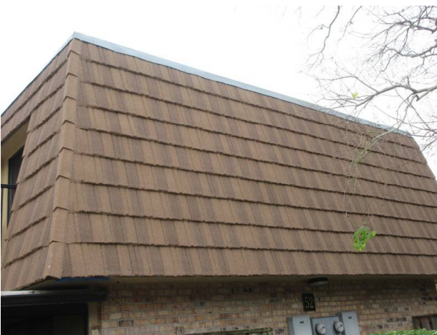
MANSARD WALLS REPLACED 2018
