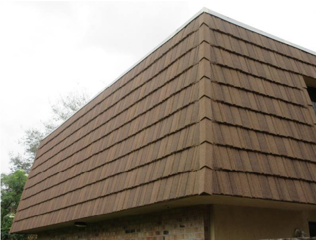
MANSARD WALLS REPLACED 2018
